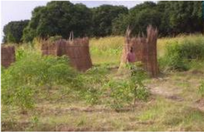
Pit Latrines used in Kaoma schools prior to the installation of Concrete Latrines by Village Water.
