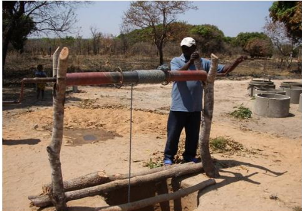
Lifting the excavated material from a hand dug well
