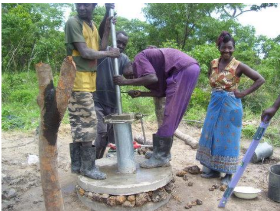
Installing pipework
