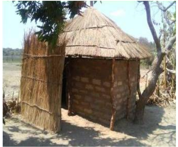
A mudbrick latrine constructed from local materials
