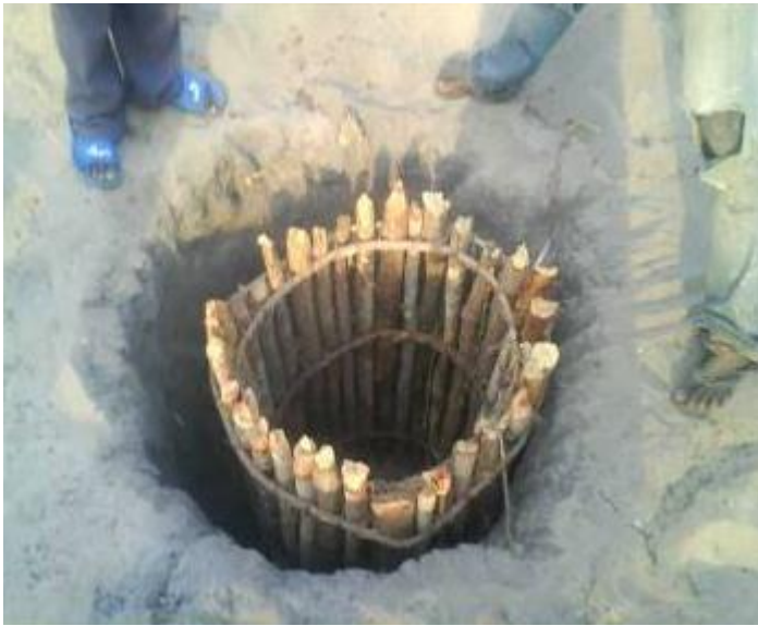
Reinforcing the walls of a pit for a latrine
