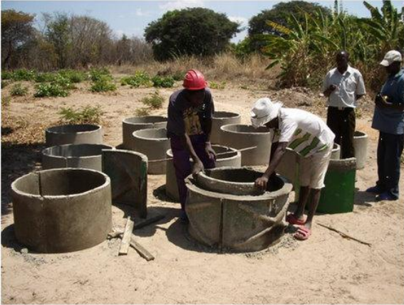
Ring moulding for the wells
