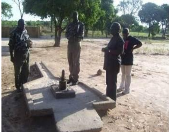
District Education Board Secretary showing Village Water staff a broken school water pump. The apron is still functioning and if the borehole still yields sufficient pure water, we will only need to replace the pump and set up a maintenance scheme as part of a WASHE programme.
